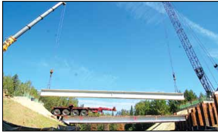
The Rez Rd. bridge construction site on Sept. 3 as the girders were put into place.
