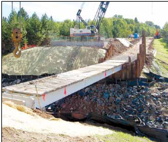
The Rez Rd. bridge construction site on Sept. 3 as the girders were put into place.
