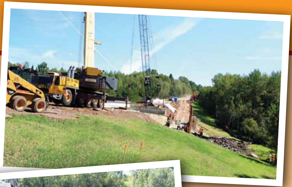
Photos from the Reservation Rd. bridge construction during the beginning of September. After the crews dug out what was left from the old culvert, they began the process of making the bridge by laying the girders across the new opening.
