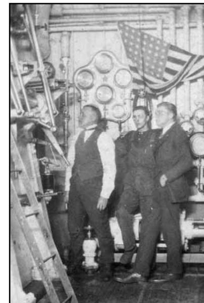
The America's engine room crew in their place of work.
